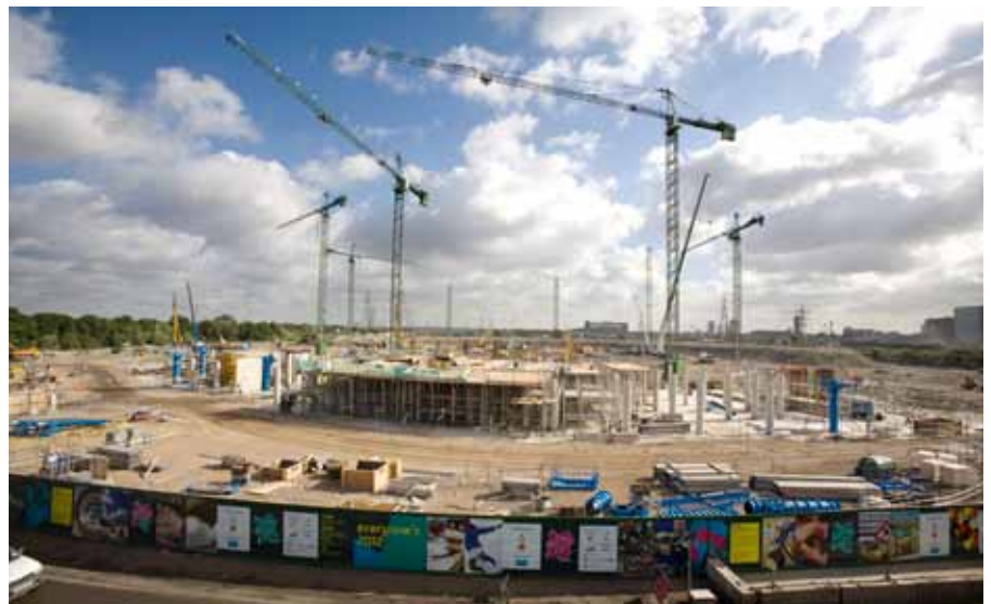
Timber is used in many different forms, including site hoarding
